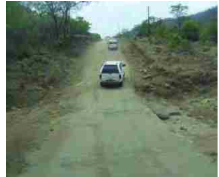
Access road to local health center submerging in rainy season (Southern Province)
